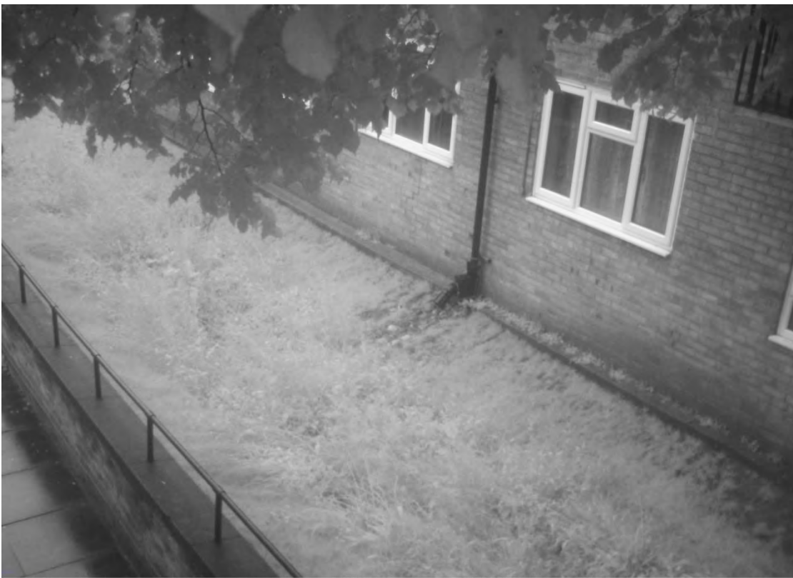
Figure 19. Time-lapse camera images from Beatrice House swale (FPC4). Images show no sign of excessive pooling in the swale i) during the period of intense rainfall or ii) following the cessation of the most intense period of the rain event.
