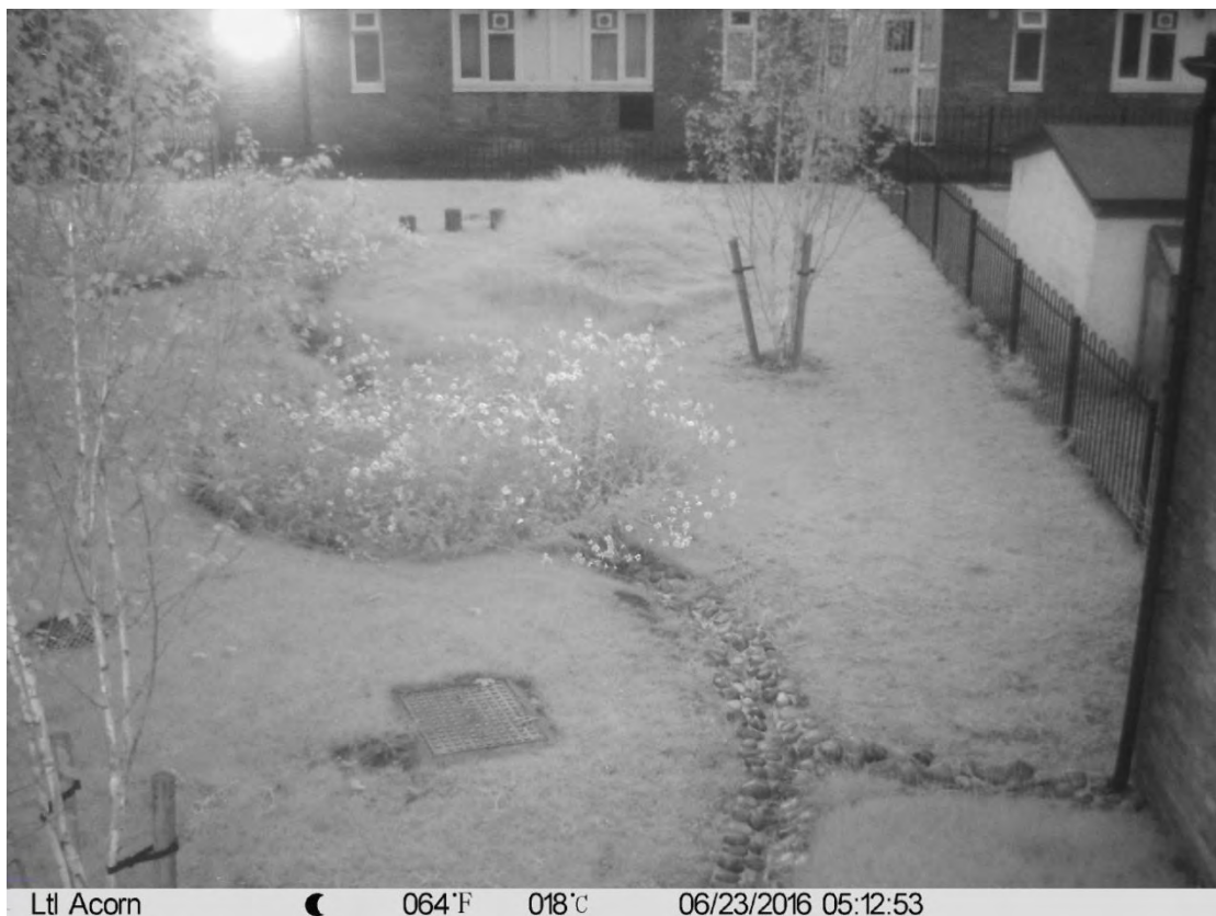
Figure 20. Time-lapse camera images from Adella House basin (FPC2). Images show no sign of excessive pooling in the basin i) during the period of intense rainfall or ii) following the cessation of the most intense period of the rain event.
