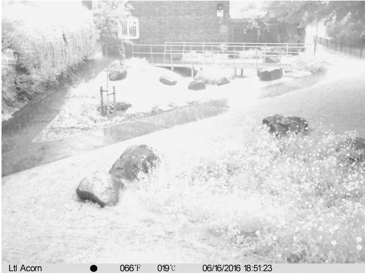
Figure 11. Time-lapse camera images from Adella House grass basin and Adella House stoney basin (FPC3). Image shows no evidence of swale filling excessively during period of highest rain intensity 18:30 to 20:00 on 16/06/2016 [32.8 mm of rain at maximum intensity of 188.8 mm/hr].
