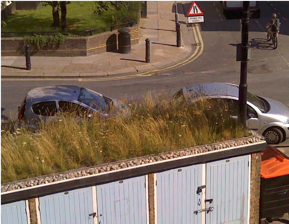
Figure 50. Photo and infrared image of pram shed roofs at Queen Caroline Estate 19th July 2016. Infrared image reveals a temperature difference of 36.0 °C between the hottest and coolest areas within the field of view. A FLIR QuickReport spotmeter was used to identify individual temperatures within the field of view. Hottest temperatures (>47 °C) were associated with the road and neighbouring paving areas. These areas were recorded as being substantially hotter than the maximum daily temperature recorded by the nearby weather station (32.6 °C). Coolest temperatures were associated with the tall vegetated areas of the pramshed green roofs (with temperatures from 33.9 °C to 35.9 °C). The roof edges were also hot (45.7 °C and 50.3 °C).
