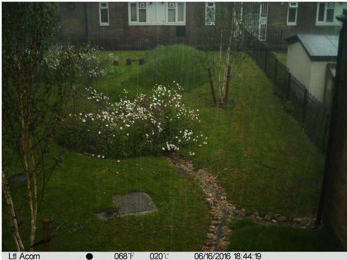
Figure 10. Time-lapse camera images from Community Hall and Sophia House basins (FPC2). Image shows no evidence of swale filling excessively during period of highest rain intensity 18:30 to 20:00 on 16/06/2016 [32.8 mm of rain at maximum intensity of 188.8 mm/hr].
