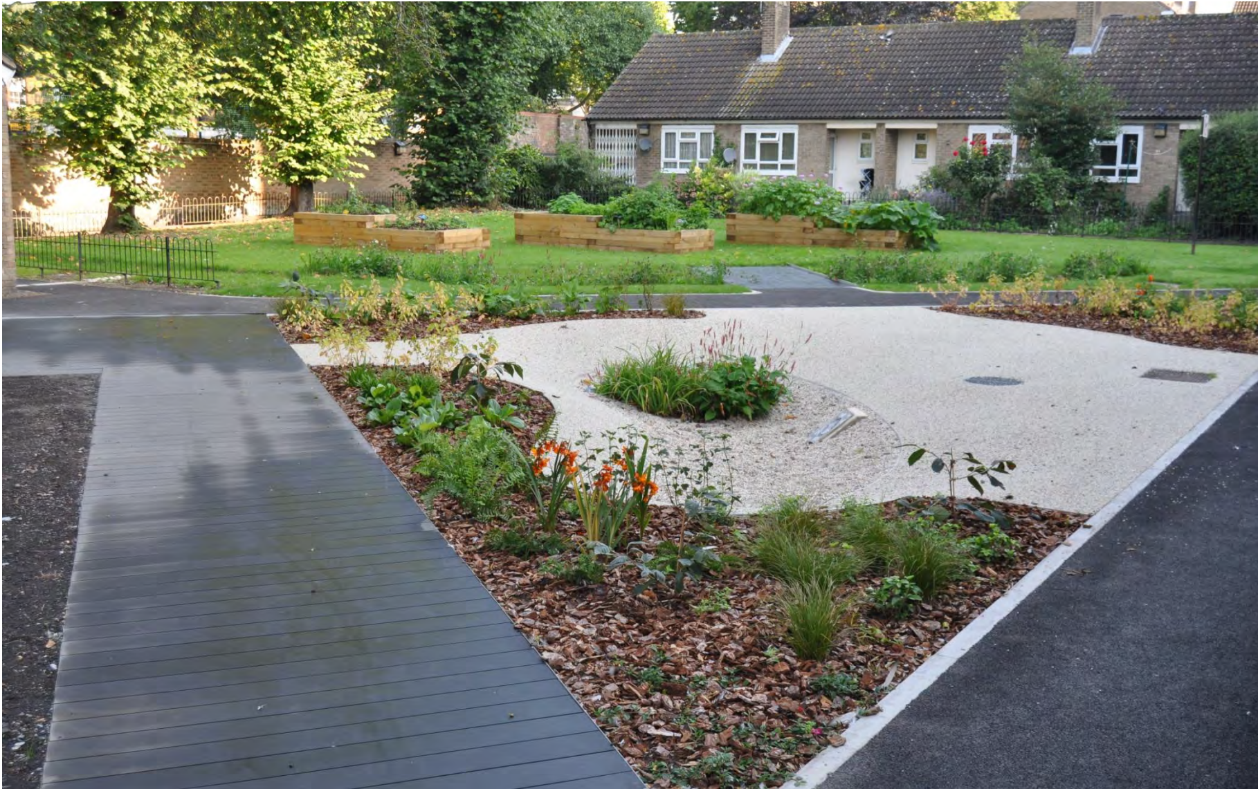
Figure 1. Green infrastructure retrofit at Queen Caroline Estate, London Borough of Hammersmith & Fulham. Raised planters, permeable pathways, ornamental planting, pollinator-friendly swales and detention basins.
