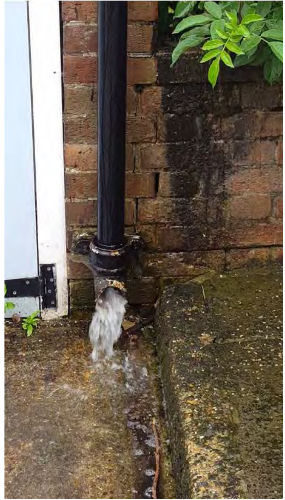
Figure 29. Queen Caroline Estate pramshed roof downpipe outflows. Images show runoff from downpipe to ground level drainage during a storm event on the 16th June 2016 for i) a pramshed with a green roof installed, and ii) a pramshed with no green roof installed.
