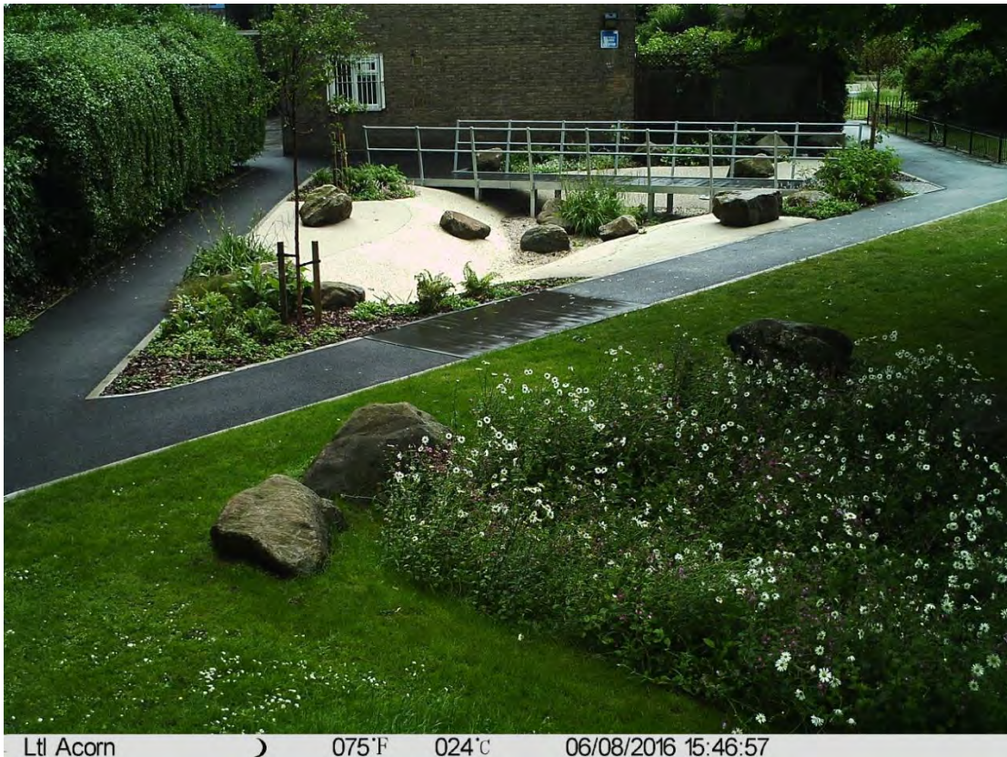
Figure 26. Time-lapse camera images from Adella House basin (FPC3). Images show no sign of excessive pooling in the basin i) during the period of intense rainfall or ii) following the cessation of the most intense period of the rain event.
