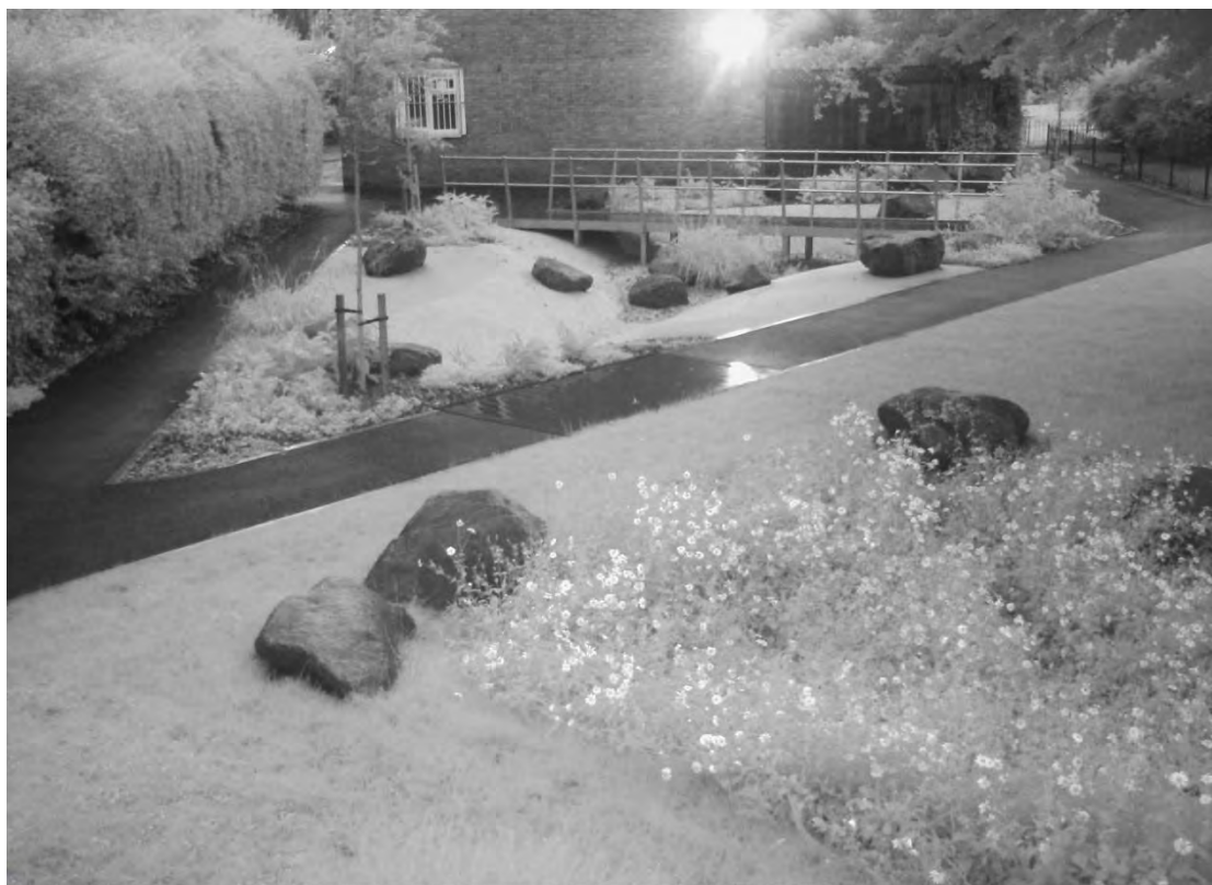
Figure 21. Time-lapse camera images from Adella House basin (FPC3). Images show no sign of excessive pooling in the basin i) during the period of intense rainfall or ii) following the cessation of the most intense period of the rain event.
