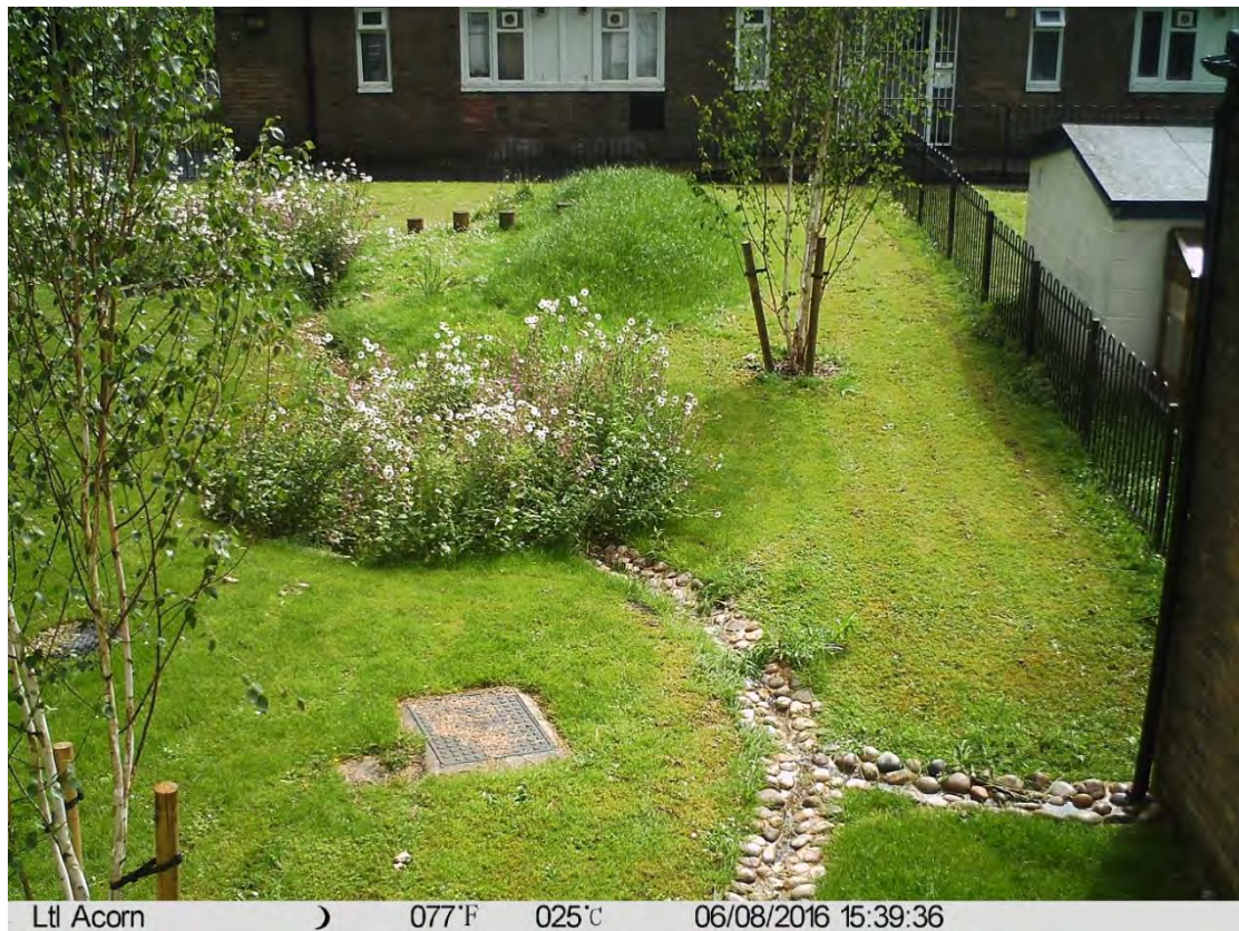
Figure 25. Time-lapse camera images from Adella House basin (FPC2). Images show no sign of excessive pooling in the basin i) during the period of intense rainfall or ii) following the cessation of the most intense period of the rain event.
