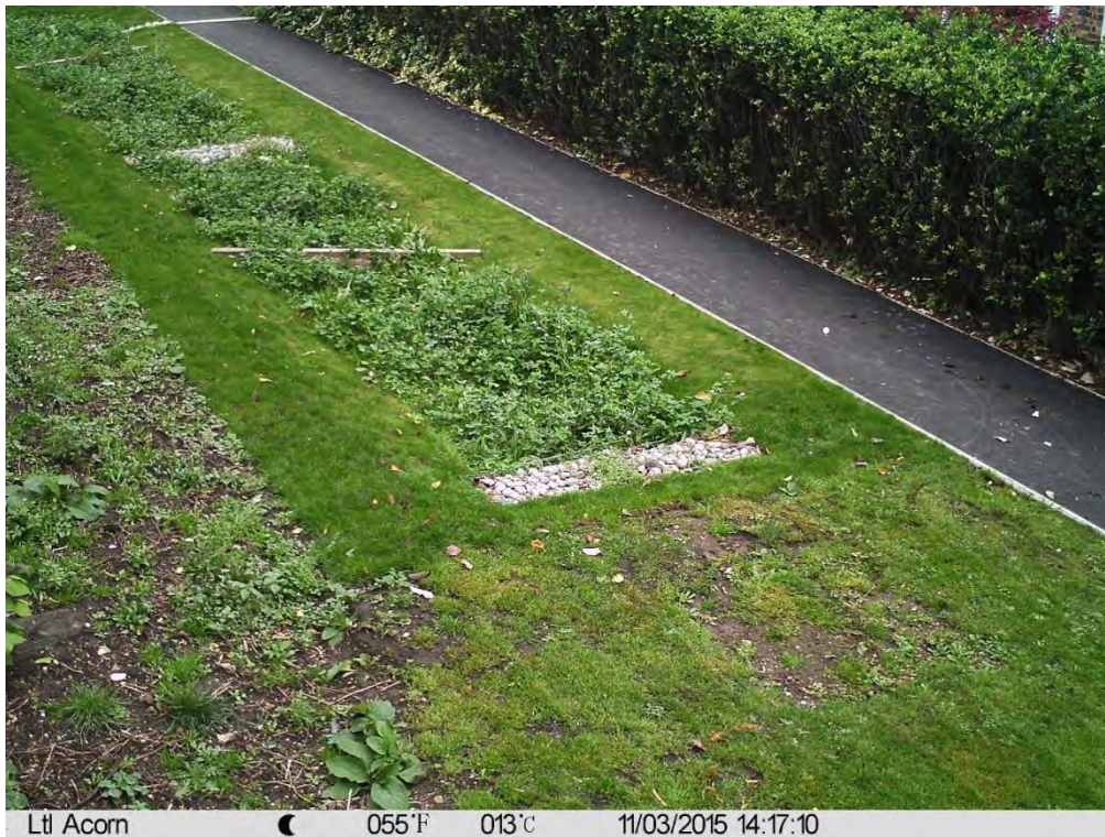
Figure 7. Field of view of fixed-point camera (FPC1) at the rear of Alexandra House, Queen Caroline Estate, London Borough of Hammersmith & Fulham. Field of view orientated to capture the lower end of the swale to monitor infiltration rates and storage capacity exceedance.
