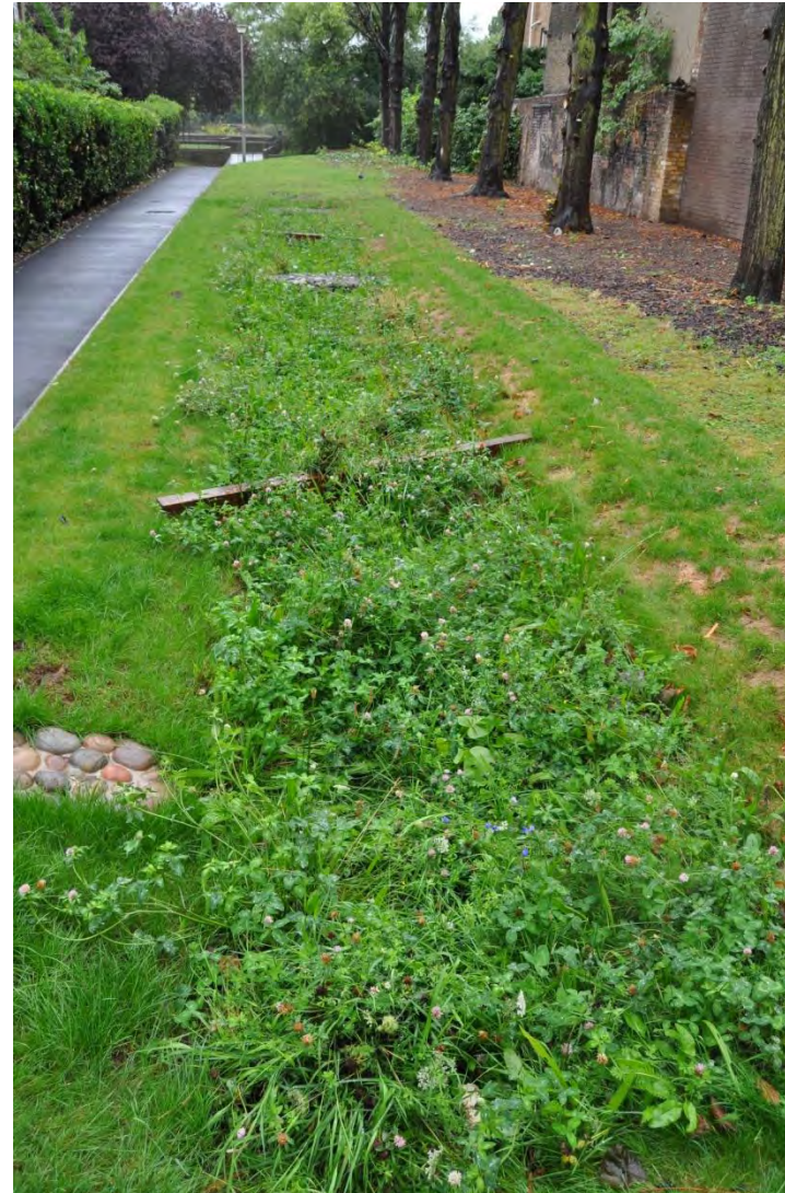
Figure 42. Alexandra House swale during a heavy rain event on the 24th August 2015. Images show i) water from Alexandra House roof being channelled into the swale; ii) no pooling at the end of the swale; iii) no pooling around the inlet to the swale.
