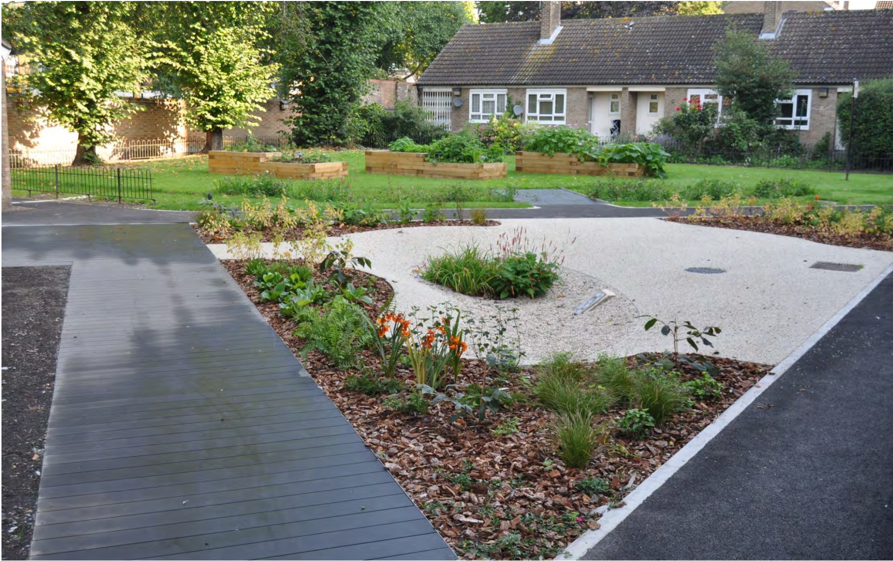
Figure 1. Green infrastructure retrofit at Queen Caroline Estate, London Borough of Hammersmith & Fulham. Raised planters, permeable pathways, ornamental planting, pollinator-friendly swales and detention basins.
