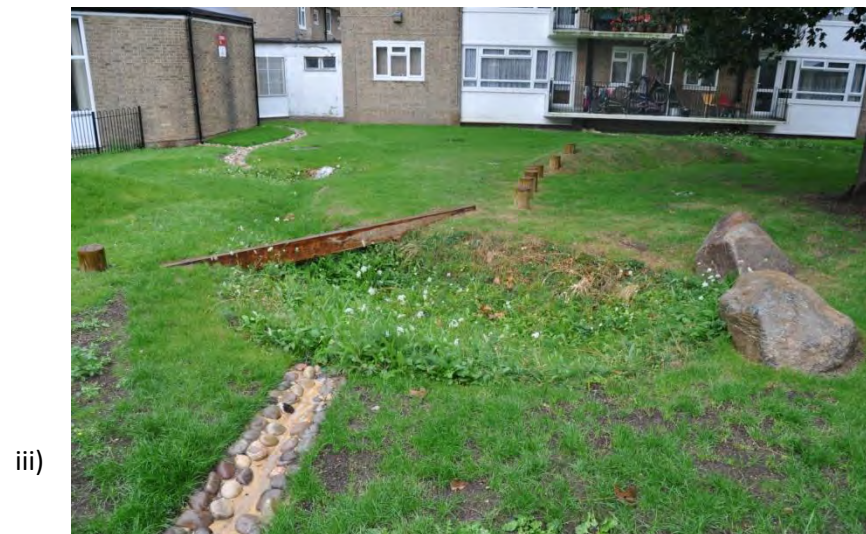
Figure 44. Sophia House basin during a heavy rain event on the 24th August 2015. Images show i) water from Sophia House roof being intercepted before entering the storm drains; ii) intercepted rainwater being diverted into basin; iii) & iv) no evidence of pooling in the basin.
