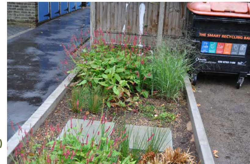
Figure 39. i) Water pooling at the entrance to the rain garden at Richard Knight House during a heavy rain event on the 24th August 2015. ii) The majority of the rain garden showing no pooling due to infiltration
