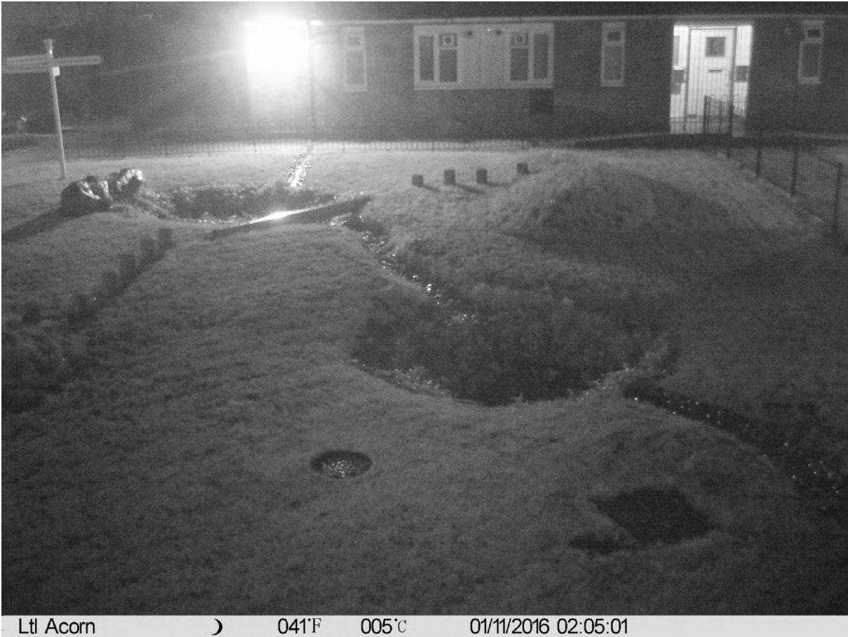
Figure 24. Time-lapse camera images from Community Hall and Sophia House basins (FPC2). Image shows no evidence of basins filling excessively during period of highest rain intensity 2am to 2:30am on 11/01/2016 [3.6 mm of rain at maximum intensity of 57.6 mm/hr].
