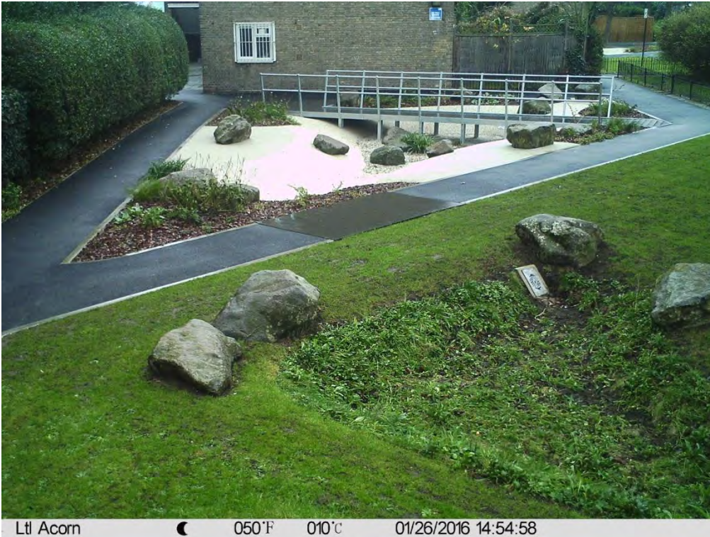
Figure 9. Field of view of fixed-point camera (FPC3) at the rear of Adella House, Queen Caroline Estate, London Borough of Hammersmith & Fulham. Field of view orientated to capture two basins to monitor infiltration rates and storage capacity exceedance.
