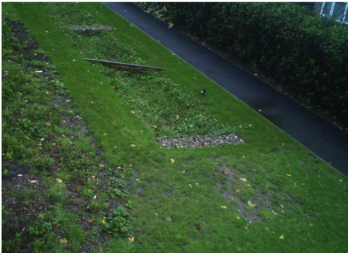
Figure 34. Time-lapse camera images from Alexandra House swale (FPC1). Images show no sign of excessive pooling in the swale i) following the period of intense rainfall or ii) towards the end of the rain event during daylight.
