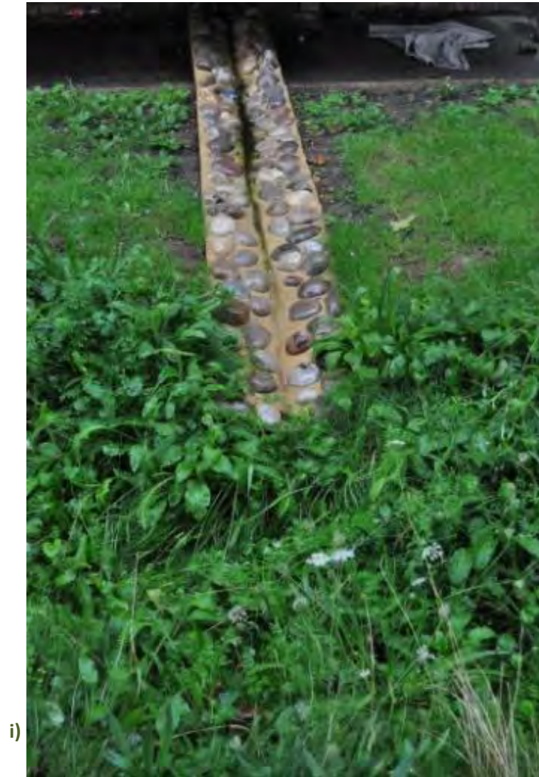
Figure 45. Adella House grass basin during a heavy rain event on the 24th August 2015. Images show i) water from Adella House roof being diverted into basin; ii) no evidence of pooling in basin; iii) no evidence of standing water near overflow.
