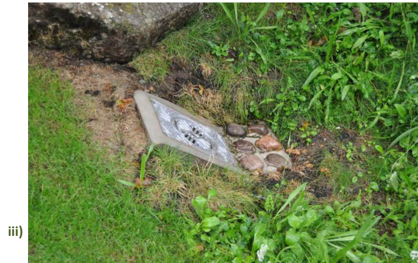
Figure 45. Adella House grass basin during a heavy rain event on the 24th August 2015. Images show i) water from Adella House roof being diverted into basin; ii) no evidence of pooling in basin; iii) no evidence of standing water near overflow.
