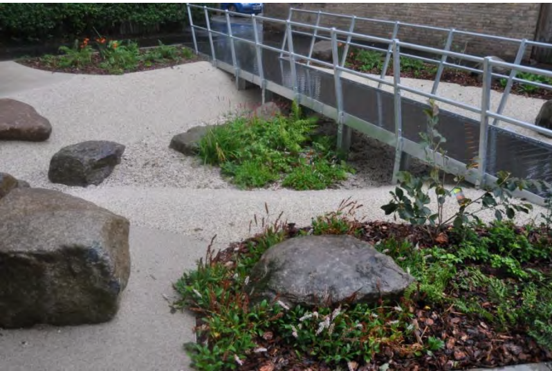
Figure 46. Adella House stoney basin during a heavy rain event on the 24th August 2015. Images show i) water from hard standing areas running into basin; ii) & iii) no evidence of pooling in basin.
