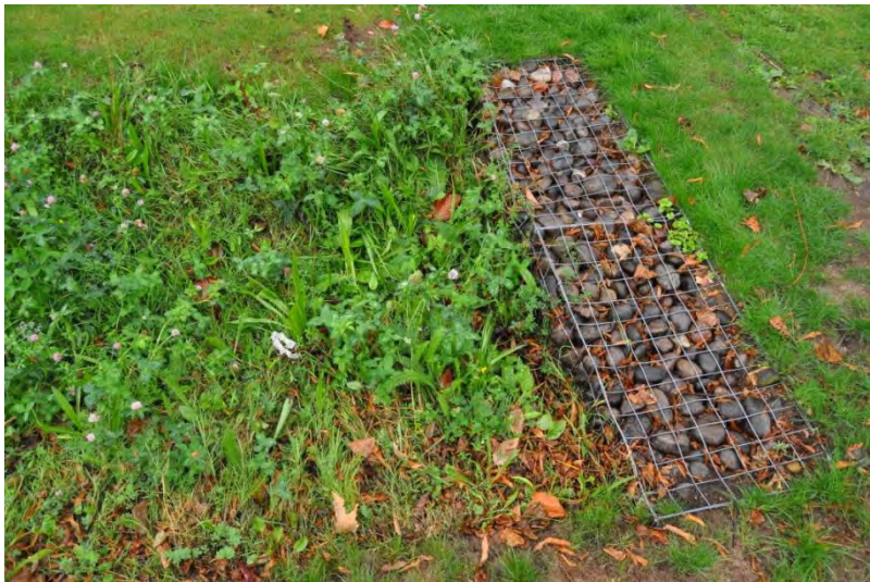
Figure 42. Alexandra House swale during a heavy rain event on the 24th August 2015. Images show i) water from Alexandra House roof being channelled into the swale; ii) no pooling at the end of the swale; iii) no pooling around the inlet to the swale.
