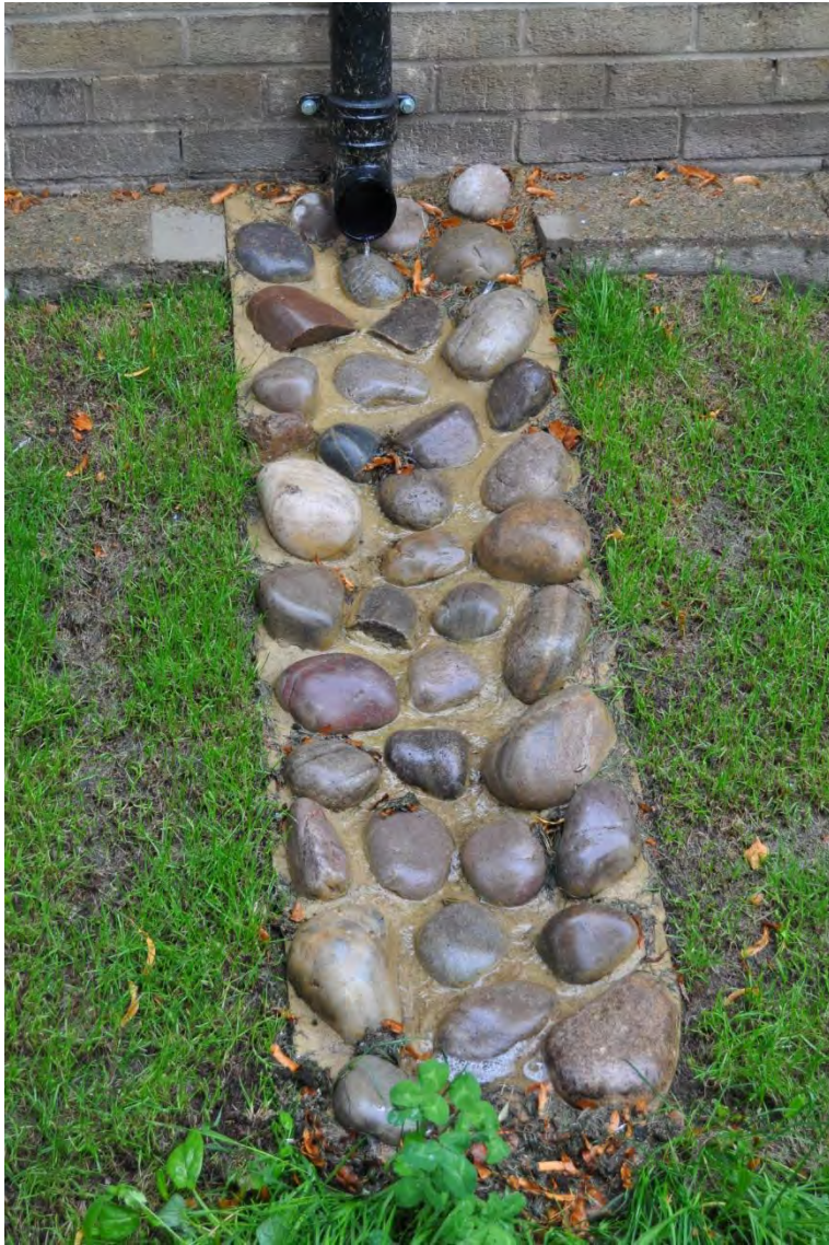
Figure 41. Beatrice House swale during a heavy rain event on the 24th August 2015. Images show i) water from Beatrice House roof being channelled into the swale; ii) pooling at the base of the swale; iii) no pooling around the outlet indicating all rainfall stored and infiltrated.
