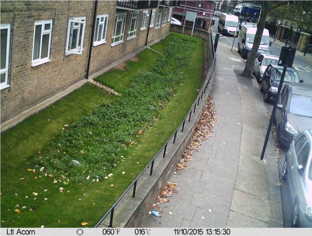
Figure 10. Field of view of fixed-point camera (FPC4) in front of Beatrice House, Queen Caroline Estate, London Borough of Hammersmith & Fulham. Field of view orientated to capture the swale whole to monitor infiltration rates and storage capacity exceedance.
