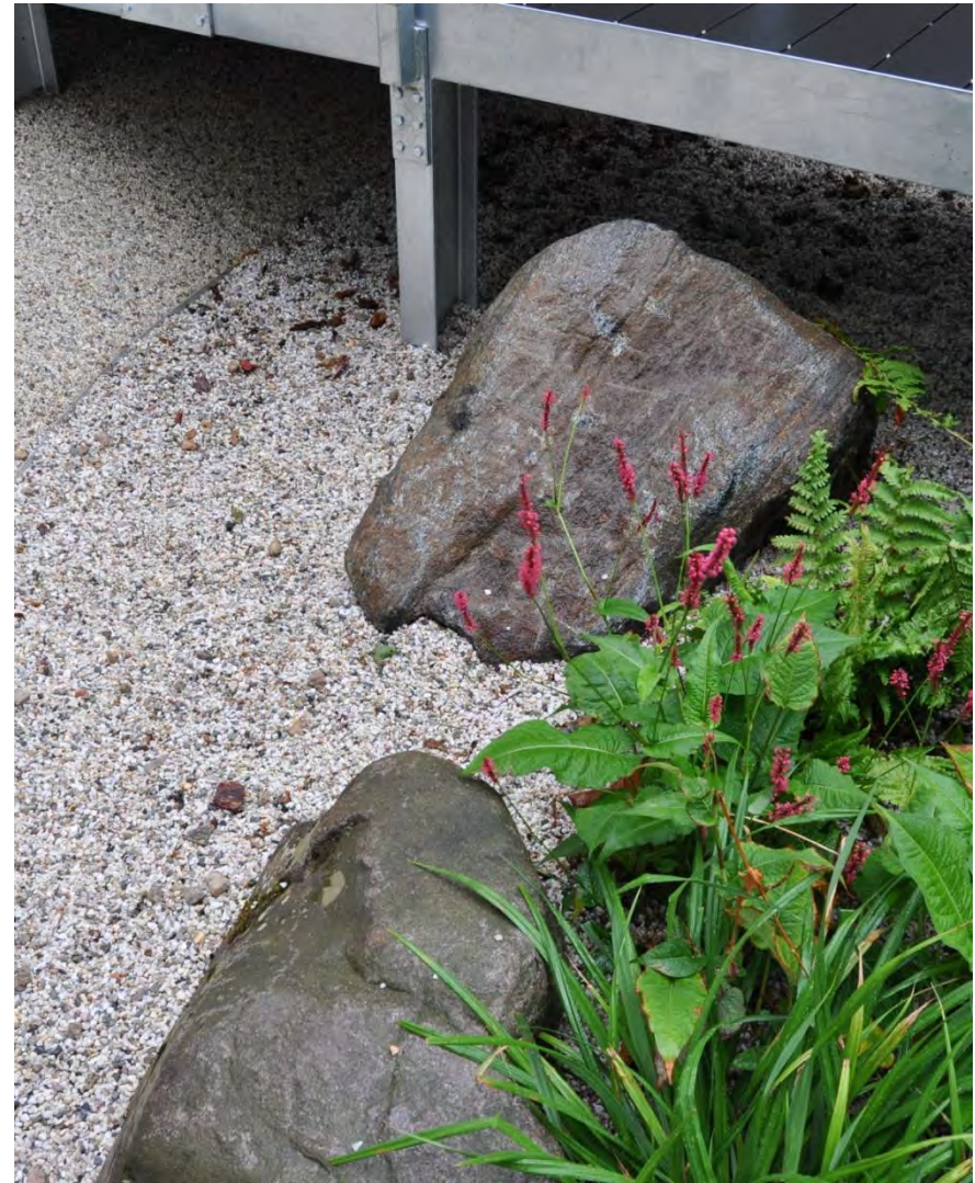
Figure 46. Adella House stoney basin during a heavy rain event on the 24th August 2015. Images show i) water from hard standing areas running into basin; ii) & iii) no evidence of pooling in basin.
