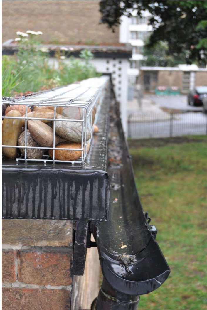
Figure 48. Pram shed green roofs at Queen Caroline Estate during a heavy rain event on the 24th August 2015. Images show i) low runoff volumes from the roof into the surrounding gutter; ii) little runoff from downpipes to ground level storm drain system.
