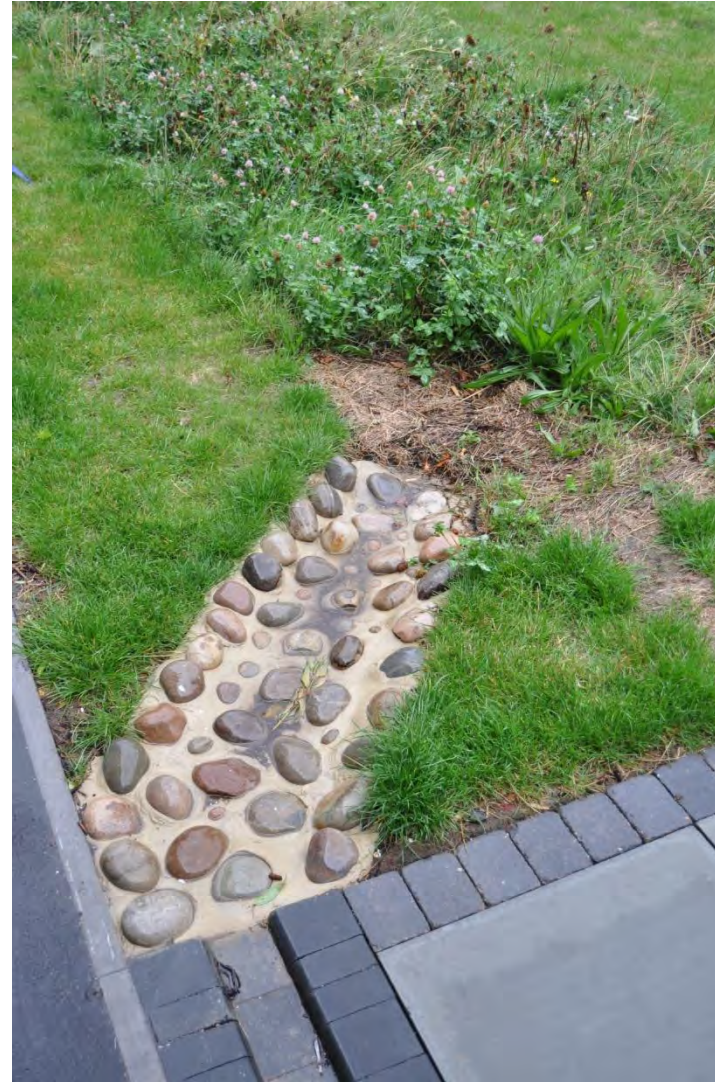
Figure 37. Water being channelled from ground-level hard standing to a swale at Richard Knight House during a heavy rain event on the 24th August 2015.
