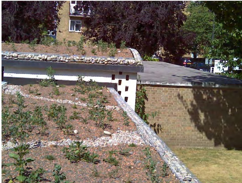
Figure 55. Photo and infrared image of pram shed roofs at Queen Caroline Estate 10th July 2015. A FLIR QuickReport spotmeter was used to identify individual temperatures within the field of view. Image showing the difference in temperatures between the green roof retrofitted pram shed roofs and the bare roof. Infrared imaging reveals temperatures from 42.5°C to 45.3°C on the bare flat roof and temperatures of 28.7°C to 57.7°C on the green roofs. Lowest temperatures on the green roof were associated with vegetated areas, highest temperatures were associated with bare substrate areas that were not yet colonised. Images were taken soon after green roof installation so vegetation was still sparse. [N.B. other images of only the bare roof recorded temperatures of 48.9 on areas hidden from the field of view of the above image].
