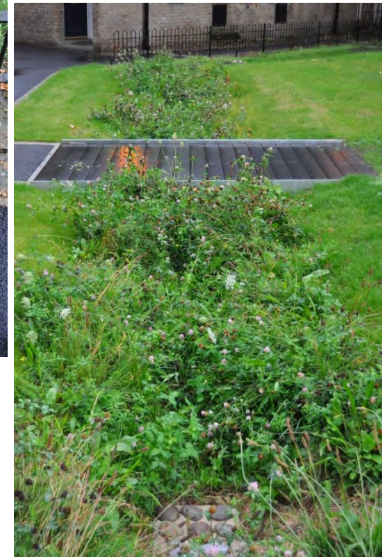
Figure 47. Phillipa House basin during a heavy rain event on the 24th August 2015. Images show i) rain from Phillipa House Roof being intercepted before entering the stormdrain system; ii) rain being channelled into Phillipa House basin; iii) no evidence of pooling near basin overflow; iii) no evidence of pooling in basin.
