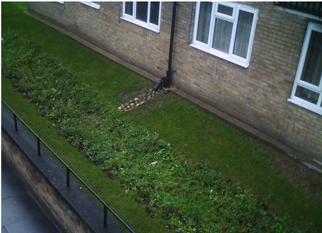
Figure 31. Time-lapse camera images from Beatrice House swale (FPC4). Images show no sign of excessive pooling in the swale i) following the period of intense rainfall or ii) towards the end of the rain event during daylight.
