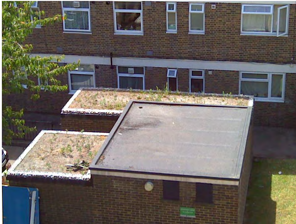
Figure 53. Photo and infrared image of pram shed roofs at Richard Knight House 10th July 2015. Image showing the difference in temperatures between the green roof retrofitted pram shed roofs and the bare roof. A FLIR QuickReport spotmeter was used to identify individual temperatures within the field of view. Infrared imaging reveals temperatures from 50.3°C to 51.5°C on the bare flat roof and temperatures of 33.6°C to 48.2°C on the green roofs. Lowest temperatures on the green roof were associated with vegetated areas and deadwood pile areas. Due to images being taken soon after roof installation vegetation was sparse. Highest temperatures on the green roofs were associated with bare substrate areas that were not yet colonised.
