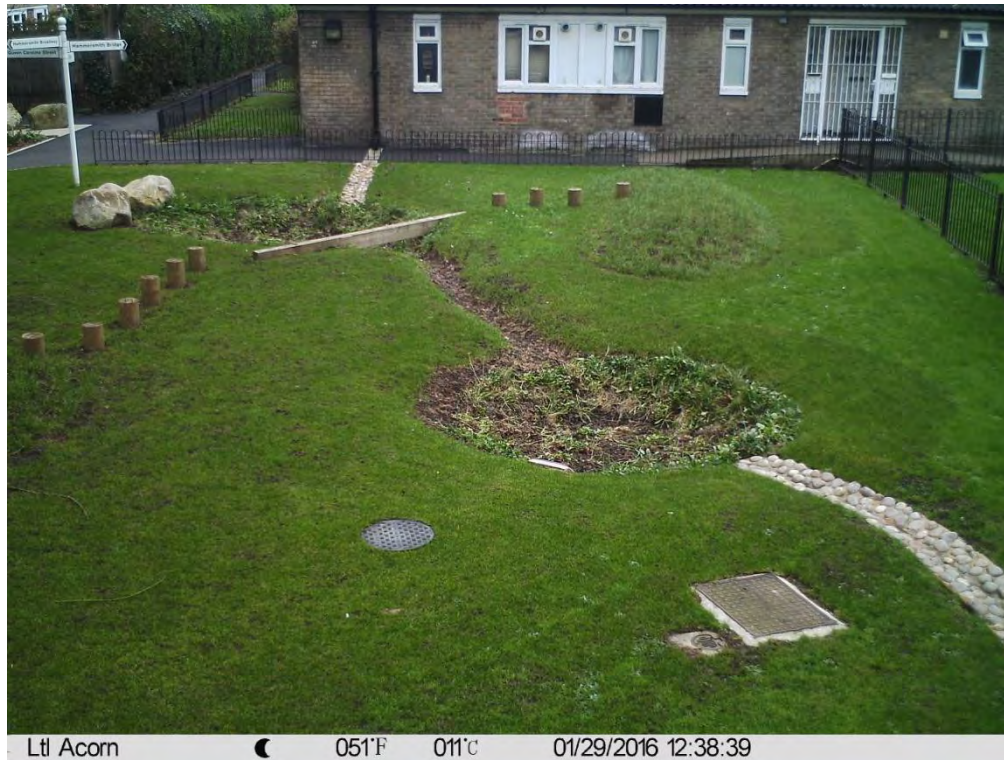
Figure 8. Field of view of fixed-point camera (FPC2) at the rear of Adella House, Queen Caroline Estate, London Borough of Hammersmith & Fulham. Field of view orientated to capture the lower basin to monitor infiltration rates and storage capacity exceedance.
